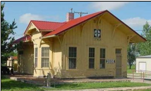
The museum with yellow paint typical of early 20th century Santa Fe depots. When the Society prepared to repaint the building in 2002, they discovered the original 1880s reddish-brown color scheme.
